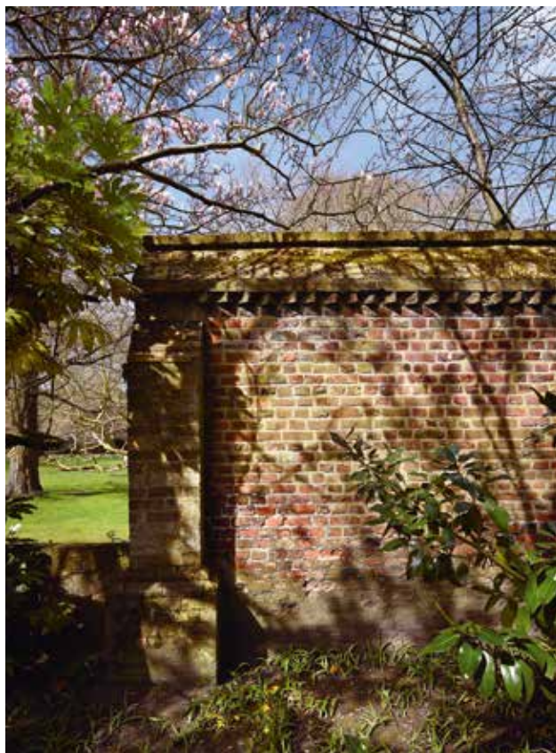
The buttress, shown at C on J B Peace's plan, marks the original south-east corner of the tennis court, although the buttress itself is of a later date.
