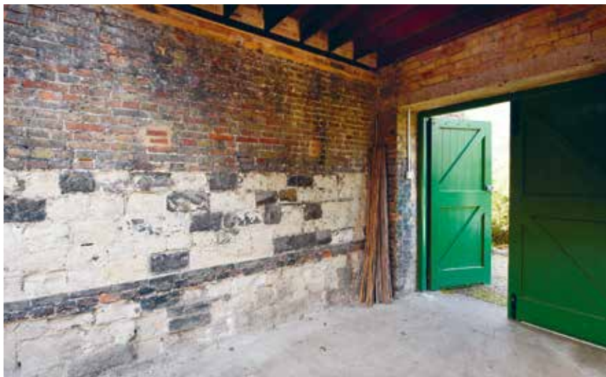
The interior of the tennis court, showing its brick, clunch and stone construction
