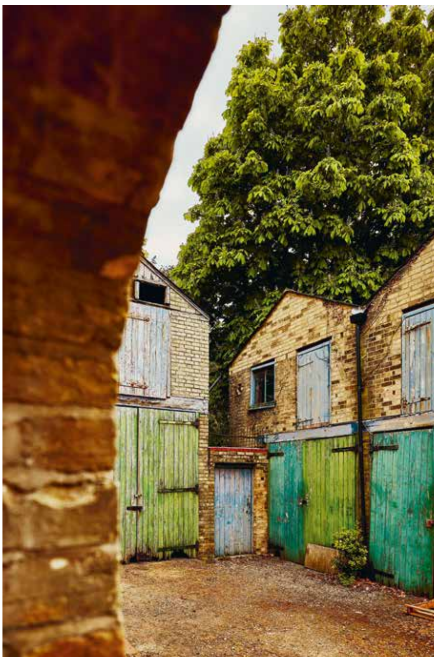
A SELECTION OF PHOTOGRAPHS SHOWING ARCHITECTURAL FEATURES OF THE COACH HOUSES
