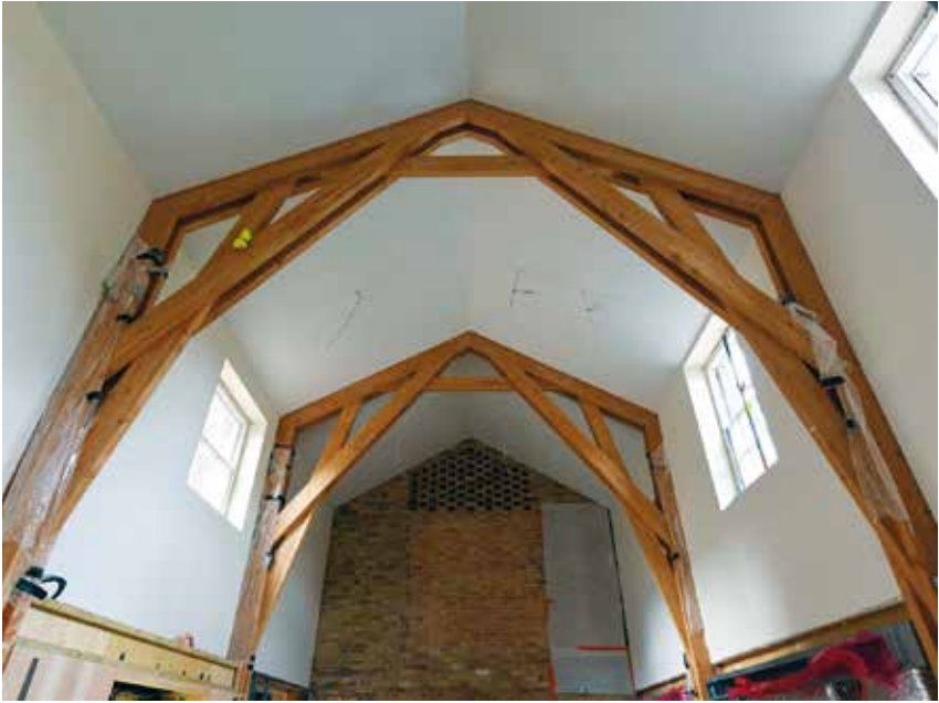
The new college bar in Furness Lodge with its scissor roof trusses
